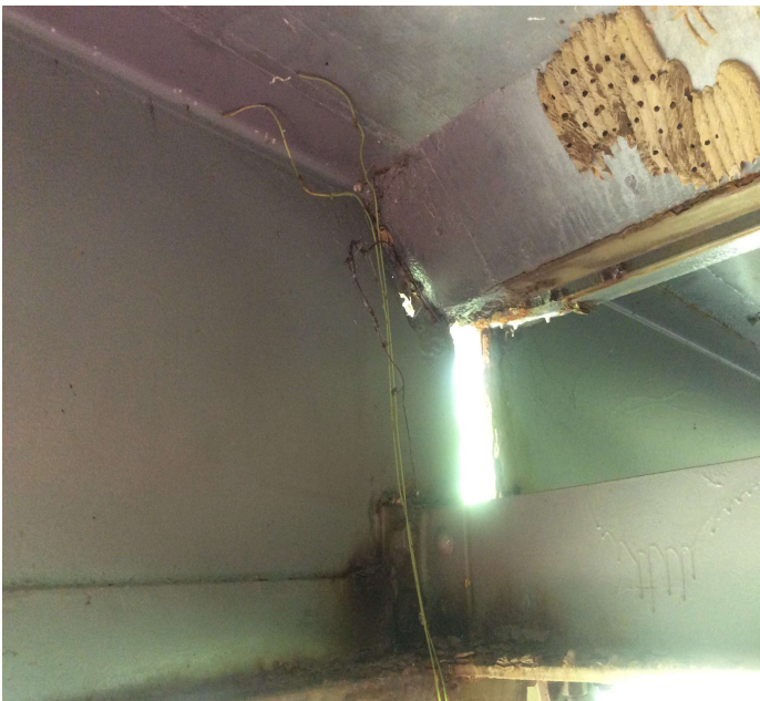
PHOTO 1 Description Span 3 Girder 5 @ Bent 3 (corrosion/hole rusted)
