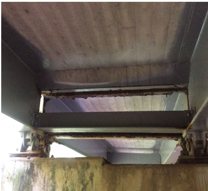
PHOTO 3 Description Girders 1-2 @ Bent 2 (corrosion)
