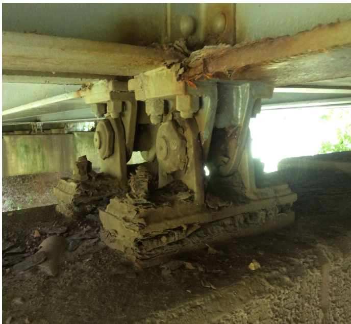
PHOTO 1 Description Bearings 4A & 4B @ Bent 3 (corrosion)
