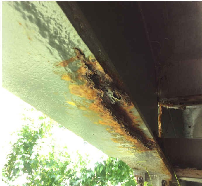
PHOTO 1 Description Span 3 Girder 5 @ Bent 3 (corrosion of bottom flange)
