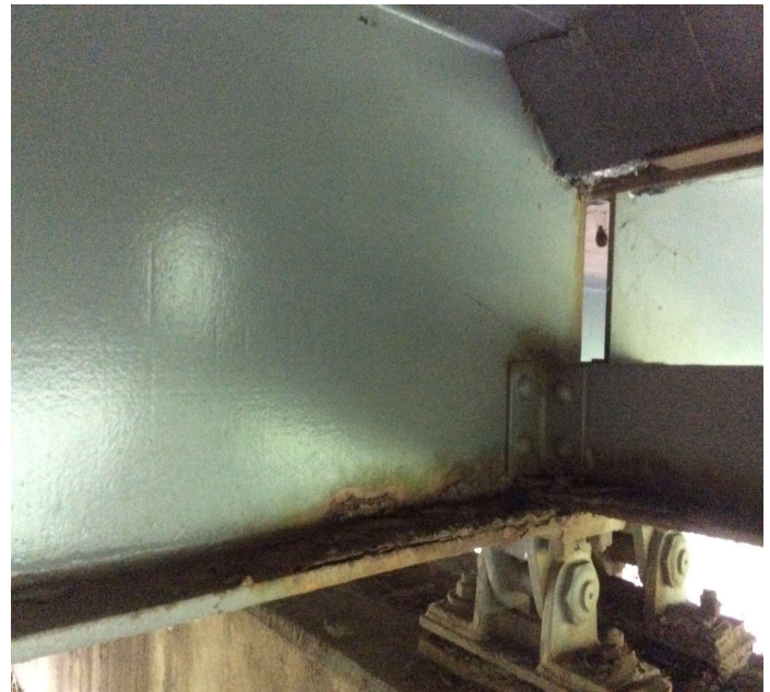
PHOTO 2 Description Span 3 Girder 2 @ Bent 3 (corrosion)
