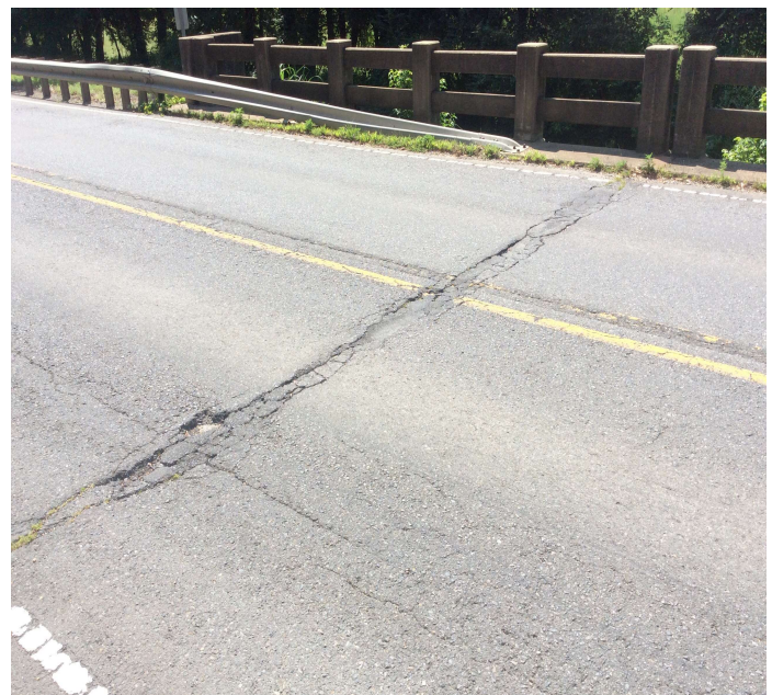
PHOTO 2 Description Wearing surface - Bent 3 (potholes)
