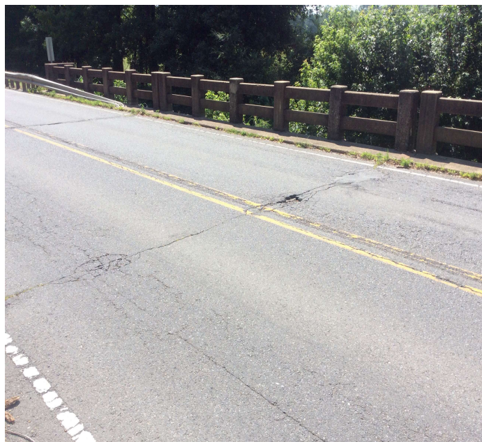
PHOTO 1 Description Wearing surface - Bent 2 (potholes)
